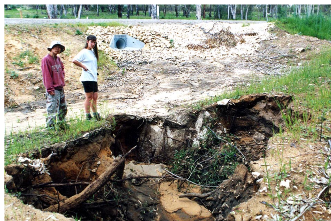
Local speleologists examining a subsidence in a new development caused by runoff from a local road.
